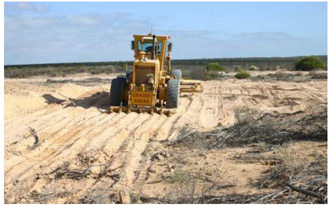
Figure 4. Large machinery such as graders can be used for site preparation including ripping, especially at mine sites and quarries. (Photo: L. Commander)
