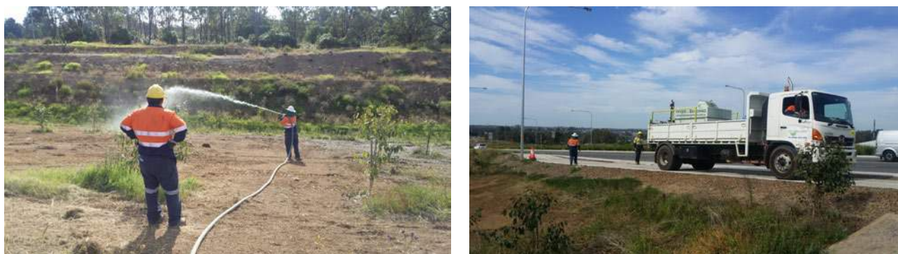
Figure 11. Hydroseeding of road batters. (Photos: P. Gibson-Roy)
