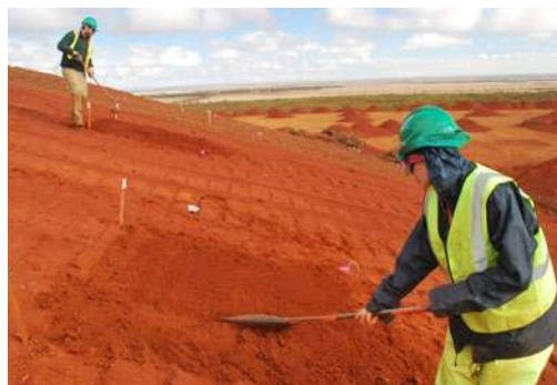
Figure 3. Raking can be used to break the surface crust, especially at a small scale, to improve soil to seed contact and prevent seed removal by wind or water. (Photos: L. Commander)
