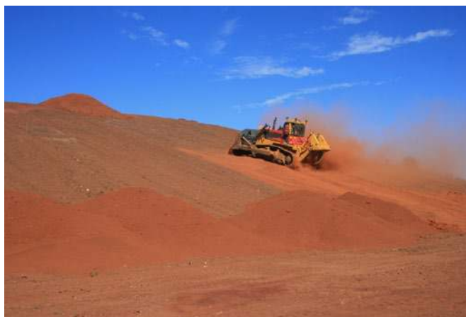
Figure 13. Spreading topsoil on a waste rock dump slope at a mine site. (Photo: L. Commander)
